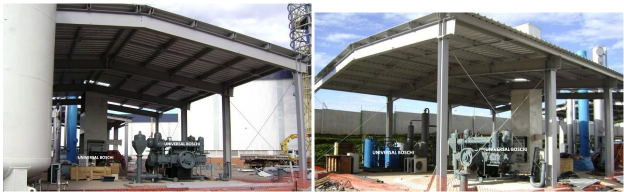
Erection of UBL 150 at Metasa Steel Plant in Brazil
