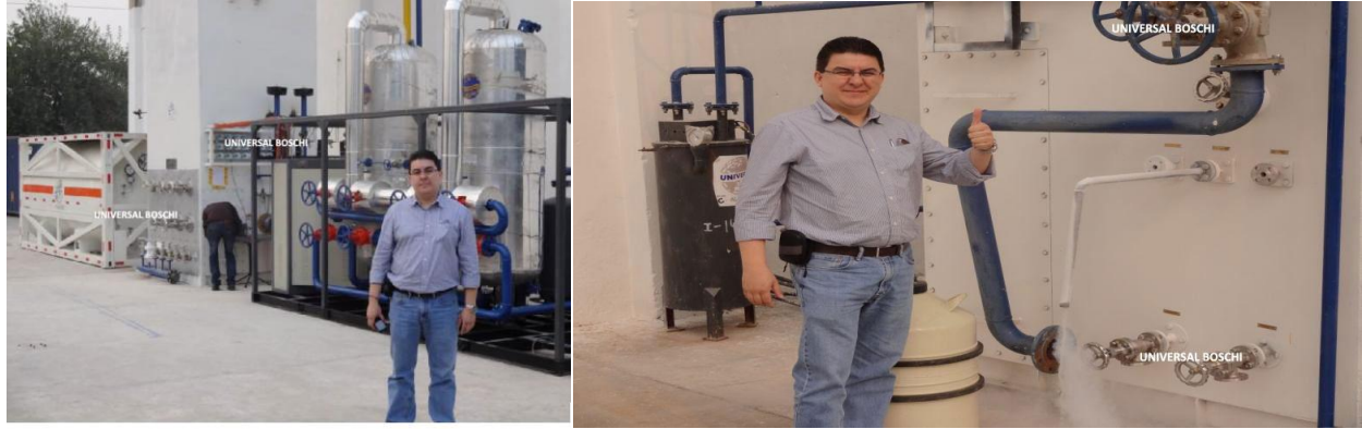
Liquid Oxygen Plant for REPSOL Oil and Gas Company (Mr. Julio after Successful Test Run of UBTL-50)
